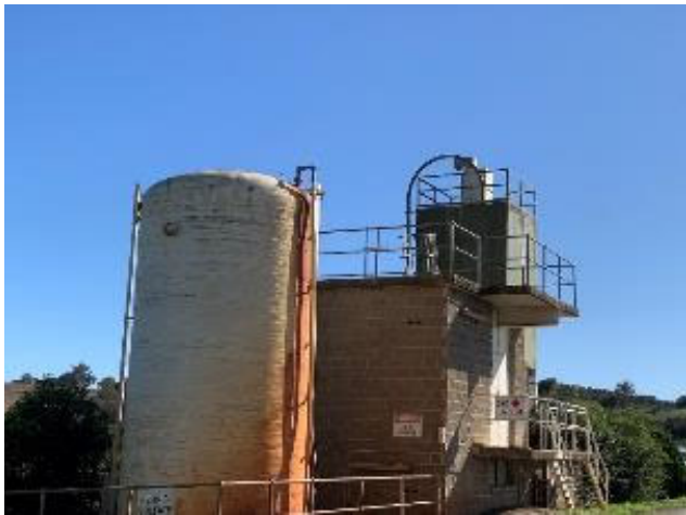
Photograph 2.5: Chemical storage on site
